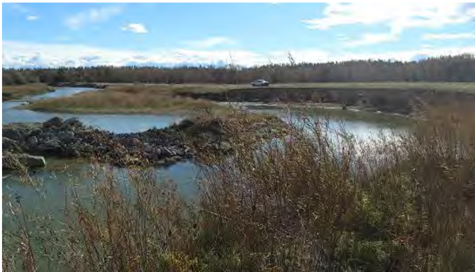
10/19/2016 Diversion broken apart and being removed, channel still flanking site.
