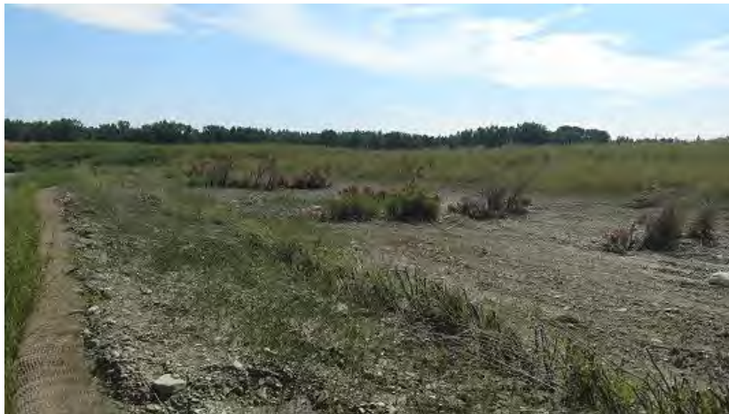
July 26th, 2017 showing the lifts, willow trench behind lift and willow with conifer cuttings perpendicular to flow in the bench
