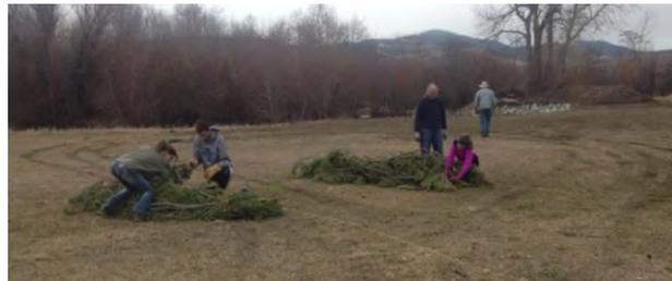
Then conifers, bundled together in a tubular shape, are staked along the edge of the water. On top of the conifer bundle willow cuttings are placed in a density of 12-15 stems per foot and on top of them a coir fabric filled with soil about one foot thick (similar to a taco shape) is laid down.
