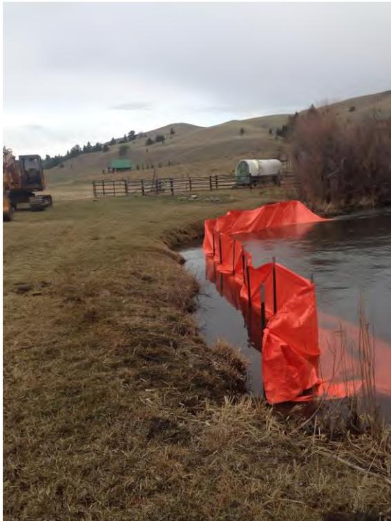
The willow soil lift is a relatively simple technique and the pictures pretty well explain the process. A machine operator excavates a terrace into the eroding bank down to the low water elevation.
