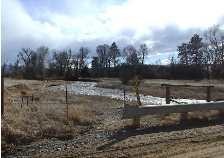
Flooding on Spokane Creek, east of Helena.
