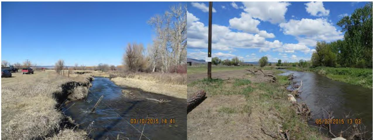
A significant amount of earthen material estimated at more than 7,000 cubic yards was moved during the project's realignment of the stream channels. These efforts to modify the stream alignment were to improve conveyance of bed load and to improve recruitment of woody riparian vegetation for erosion control as well as provide fish habitat and stream cover. Approximately 5,000 willow sprigs
