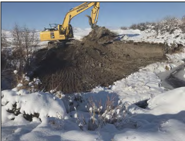
Figure 1 Excavator Opening Floodplain
