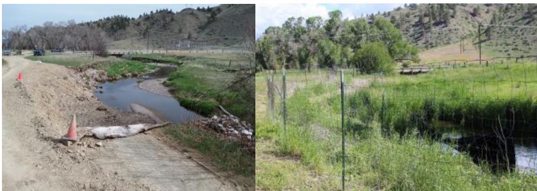
Spokane Creek Project, Before and After
